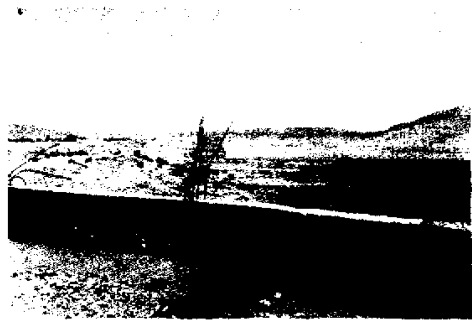
Fig. 6. Photograph showing walls across the valley to collect water, reduce floods pressure and avoid destruction.
